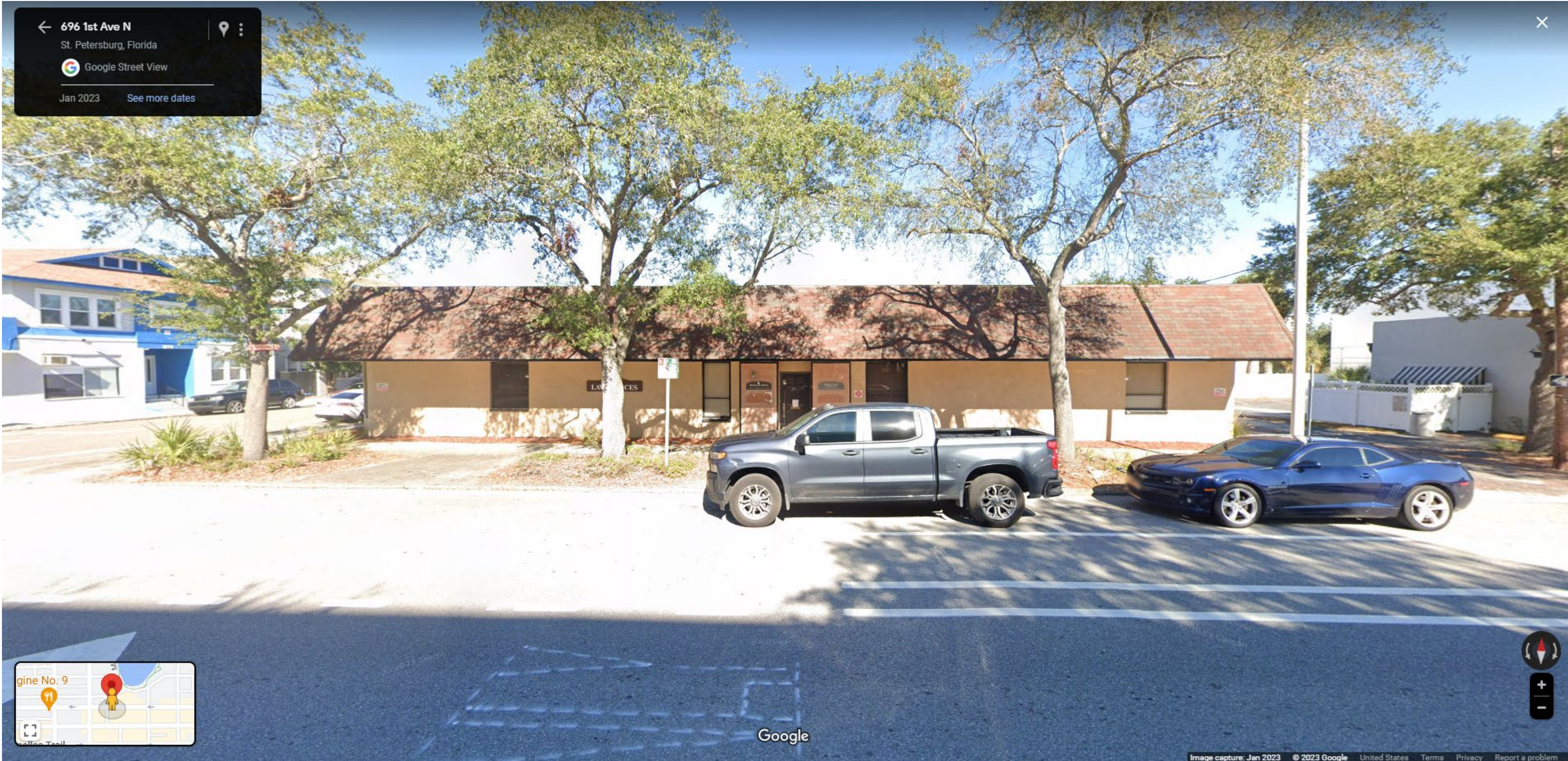
699 1 st Ave. N.- no historic features. Windows, doors and awning all appear to be non-historic later additions.
