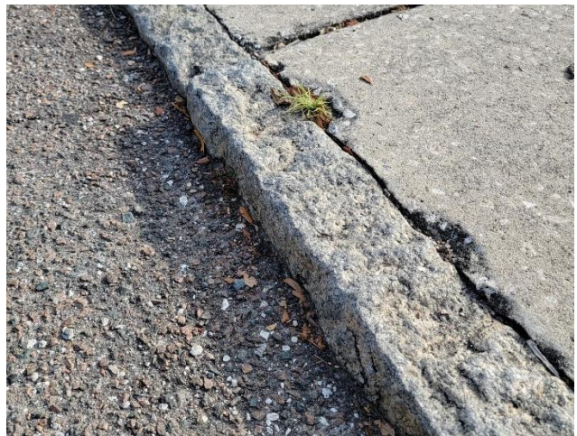
Figure 15. Example of granite curbing within the public alley and along surrounding streets.
